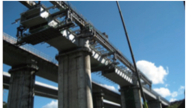
Segment Erection
