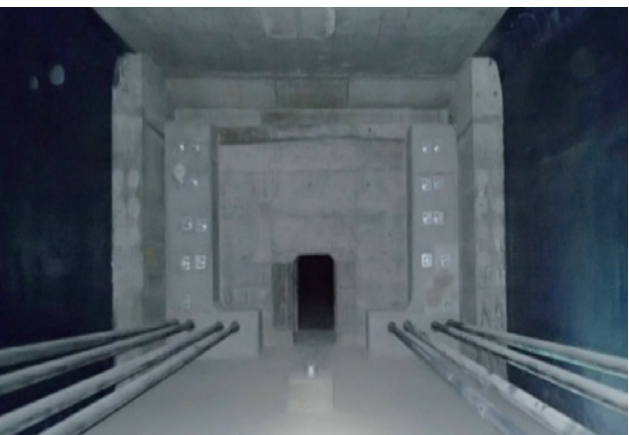
Center Hinge at Inside of Boxgirder
