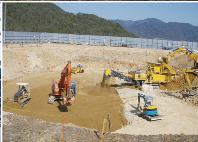
Ground Excavation for PC Tank Foundation
