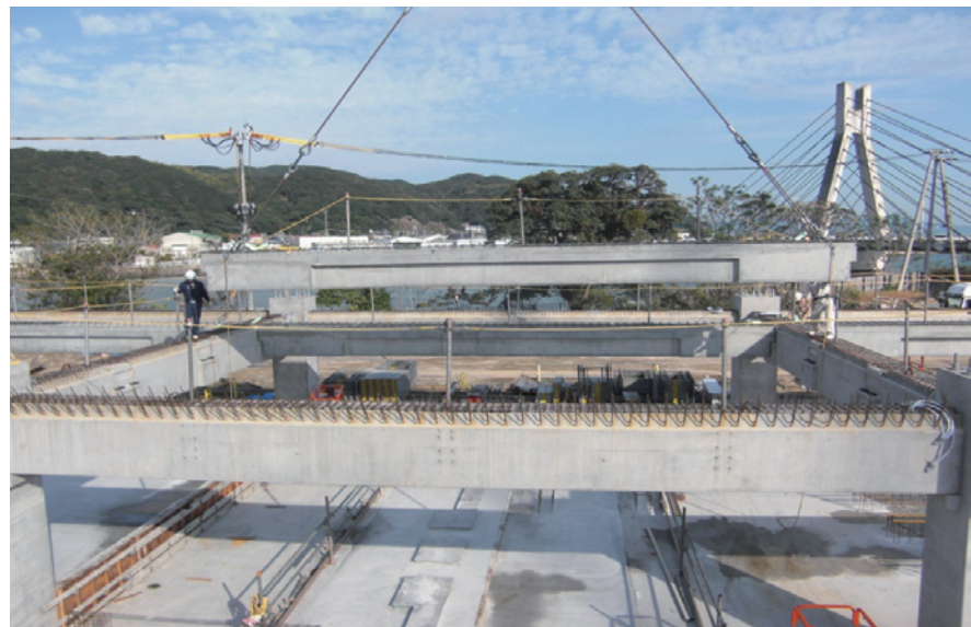
Precast Beam Installation
