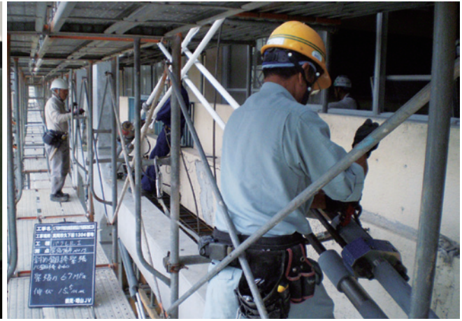
Tensioned the Skew Brace Materials
