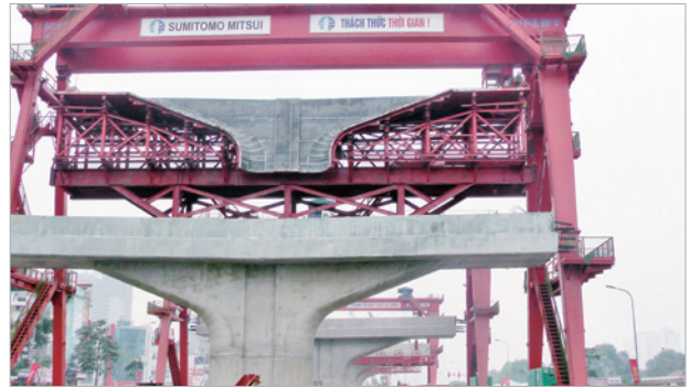
Scaffolding Falsework and Mold Form
