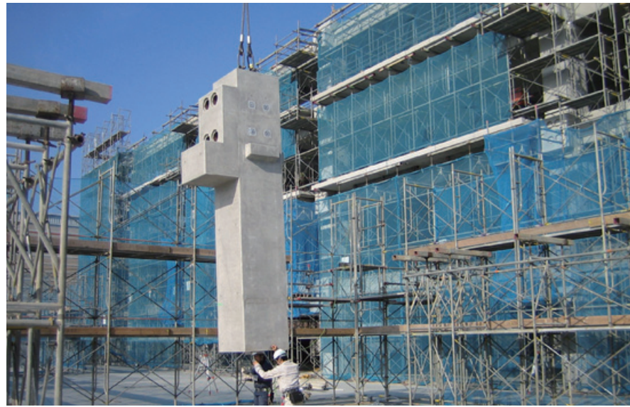
Precast Column Installation
