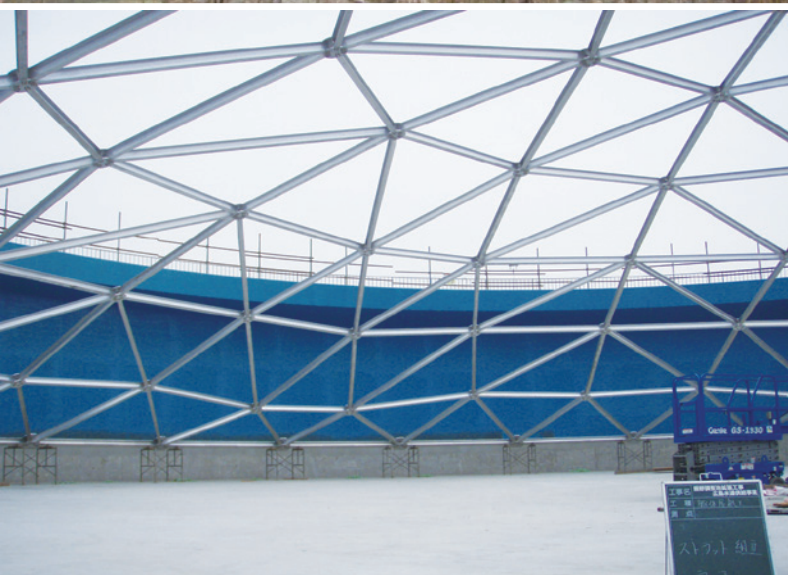
Large Scale Aluminum Dome Roof Structure
